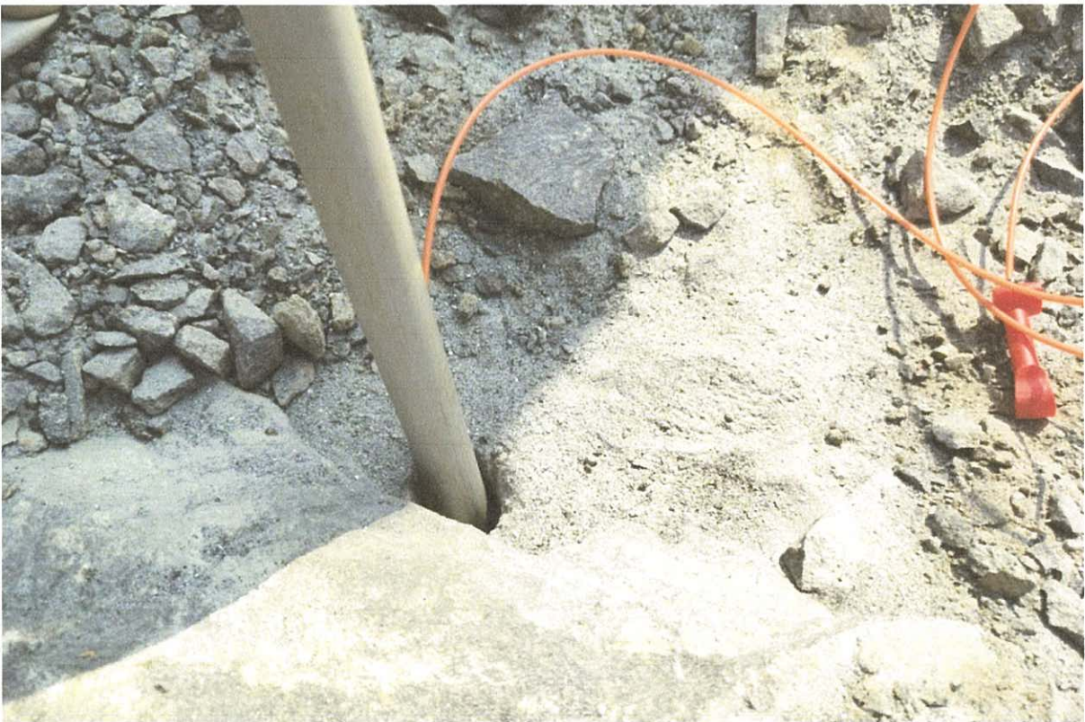
FIG. 3.9 A VIEW OF STEMMING OF THE BLAST HOLE
