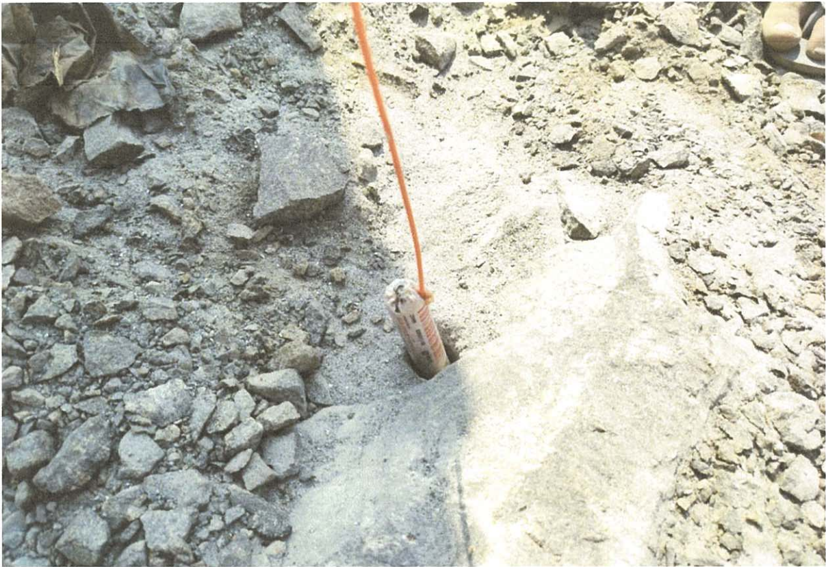
FIG.3. 8 A VIEW OF CHARGING OF THE BLAST HOLE
