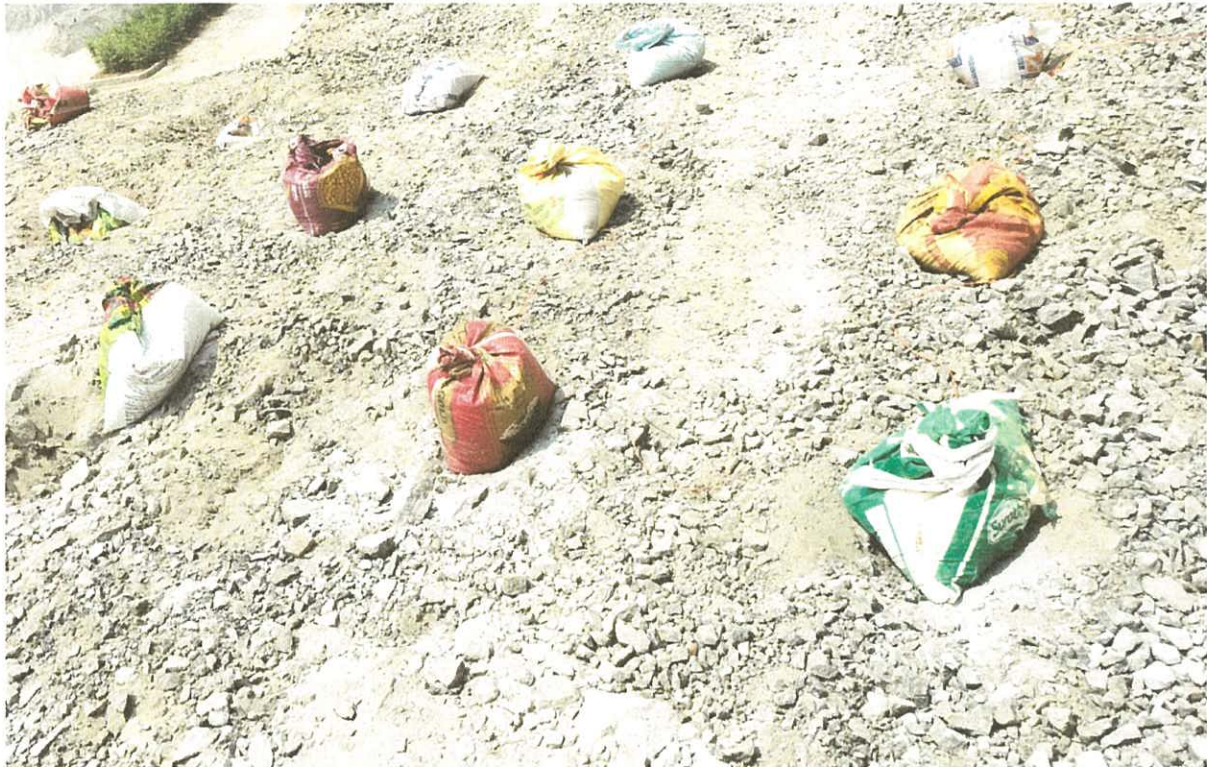
FIG. 10 MUZZLING ARRANGMENT WITH SAND BAGS
